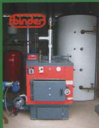
45kW Binder pellet boiler at Stockland Victory Hall, Devon Installed October 2004 by Wood Energy Ltd www.woodenergyltd.co.uk Tel: 01398 351349
